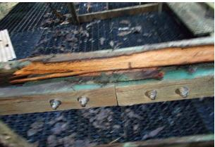
The fan deck is not the original deck. None of the seams are staggered. Plywood under the mechanical support – <u>motor side has not been replaced.</u>
