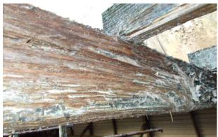
• In addition to deteriorating members in the plenum area under the fans, there is sufficient evidence of iron rot from old sprinkler hanger hardware on many of the 2 x 8, 4 x 4, and 2 x 6.
