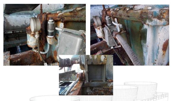
Motors and drive shafts are in good operable condition. Drive shafts had some solid build-up and should be routinely cleaned. Shaft guards are rusted and should be replaced.
