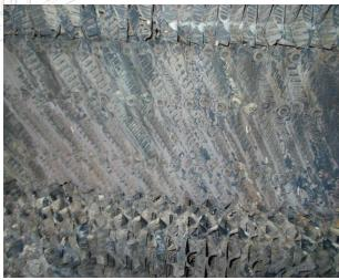
The PVC drift eliminators are in fair condition. A few areas were notices where there are gaps and/or broken modules. Estimated that there are about 12 modules per cell (1' x 8') to be replaced.
