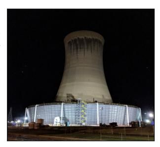
performance ArchBar fill, drift eliminators and an innovative grade level manifold system. The scope also included an all-new fiberglass canopy, bypass system and a flexible water distribution system designed to handle the tower's 384,000gpm consisting of fourteen (14) risers with individual butterfly valves to improve distribution and facilitate maintenance.
